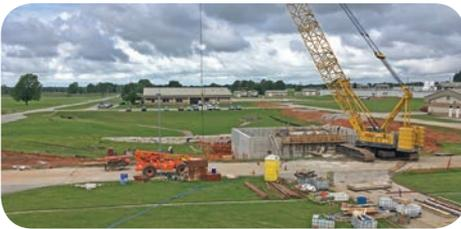
In 2018, the Filter-to-Waste (FTW) and Solids Processing Improvements Project got underway. The cost estimate for the project is \$4.8 million. The project is now more than halfway complete and is adding a recovery basin, piping, pumps, and other
