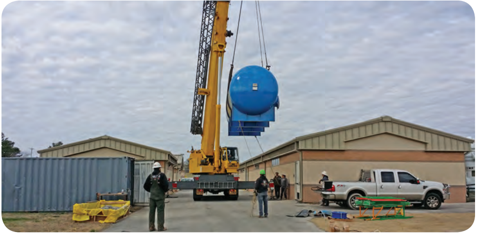
Surge Tank being lowered into Treated Water Pump Station.
