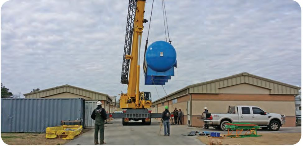
*Surge Tank being lowered into Treated Water Pump Station.*
