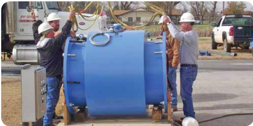
*On Nov. 19th, District staff replaced the 36-inch “magnetic flow meter” (mag meter) for the drinking water plant’s filter backwashing system. The mag meter measures the flow of water through the pipe.*
