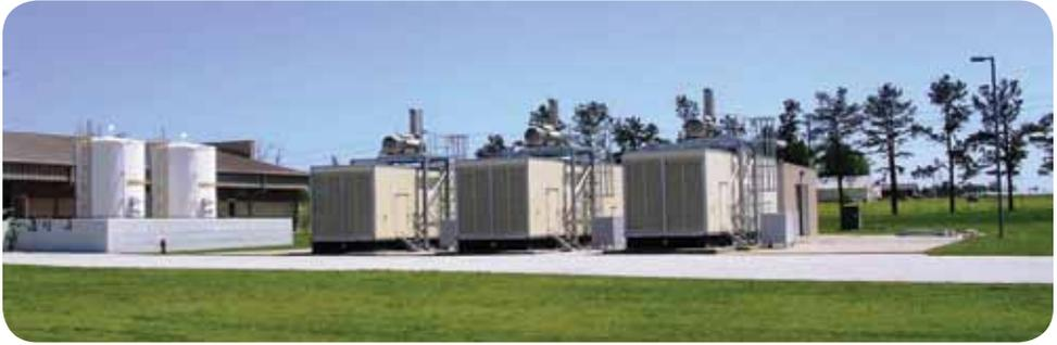
*Beaver Water District installed emission control devices on three, 2-MW diesel-powered generators.*
