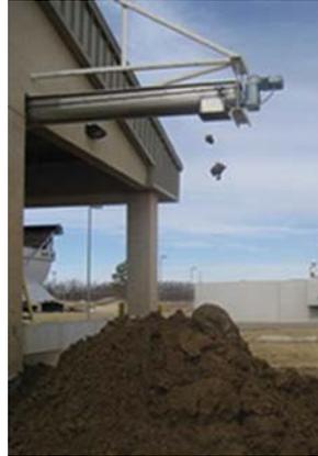
*A mixture of dirt, alum and water falls from an auger conveyor into a pile to be transferred to a dump truck at the Beaver Water District treatment plant in Lowell. (Photograph by Amy Wilson.)*
